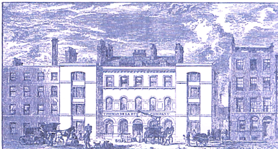
De La Rue Print Works, Bunhill Row, off Old Street, London, 1856
