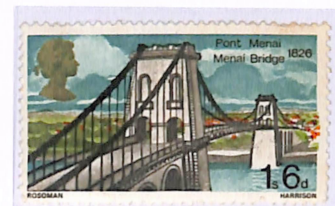
Wrought and Cast Iron Use in Bridge Construction: Menai Bridge
